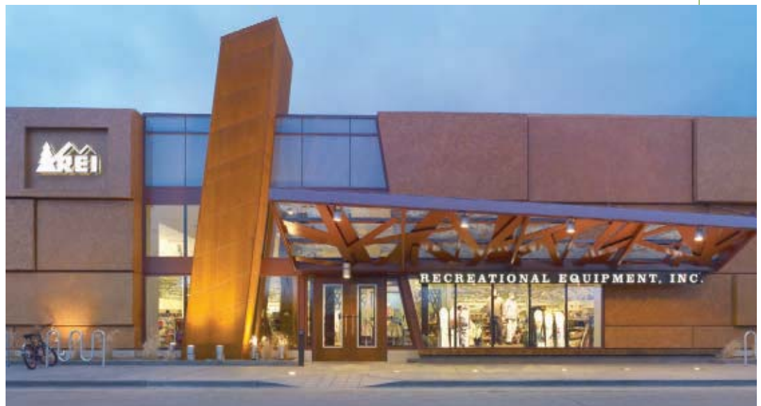
A solar hot-water system at REI’s Boulder, Colo., location will meet 70% of the store’s needs.
